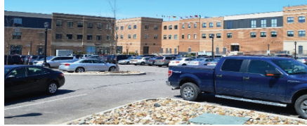
(Top) Haymaker Parkway, between Water Street and S. Depeyster Street across from the Fire Station circa 2009
